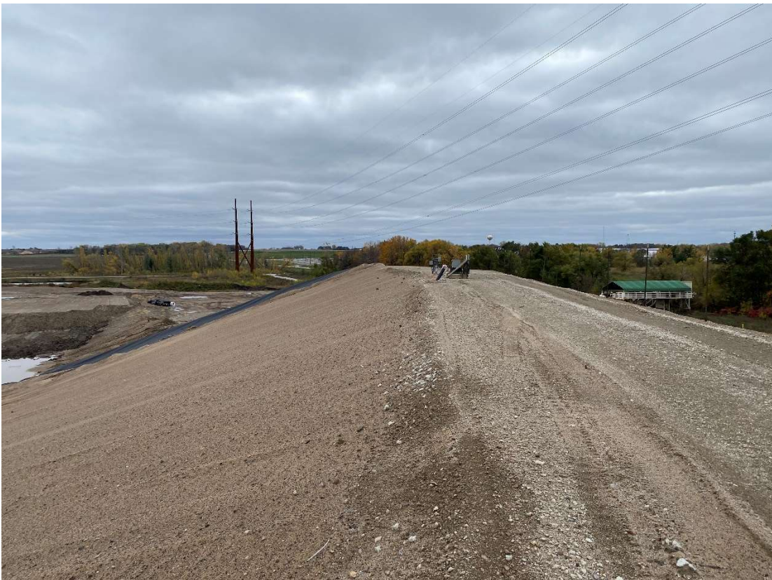
Location 14 – Cell 6, interior top of berm, looking south
