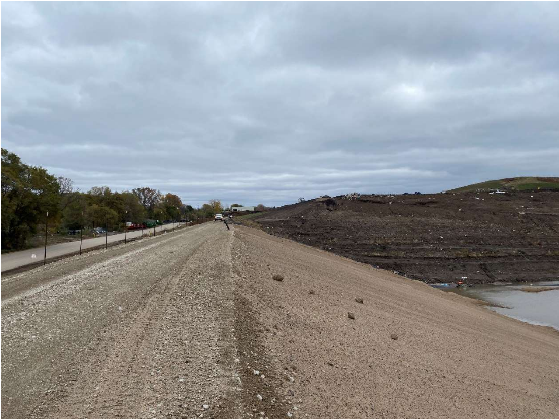
Location 14 – Cell 6, interior top of berm, looking north
