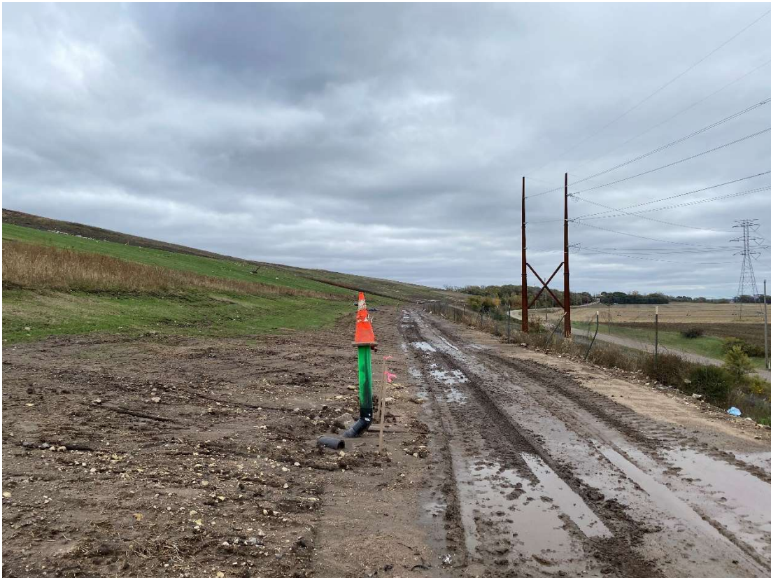
Location 7 – Cell 6, toe of southern waste slope, looking east
