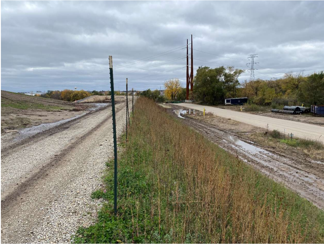
Location 15 – Cell 6 midpoint of northwestern outer berm, looking southwest
