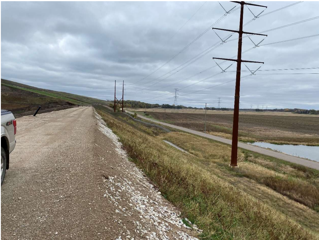
Location 8 – Cell 6, exterior of southern landfill berm, looking west
