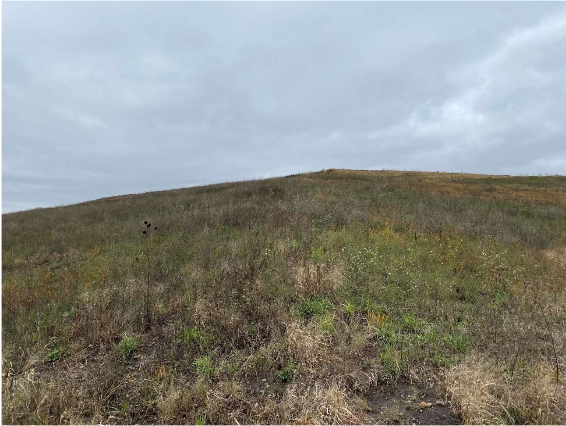
Location 5 – Looking Northwest, at Phase 3 Liner Limit
