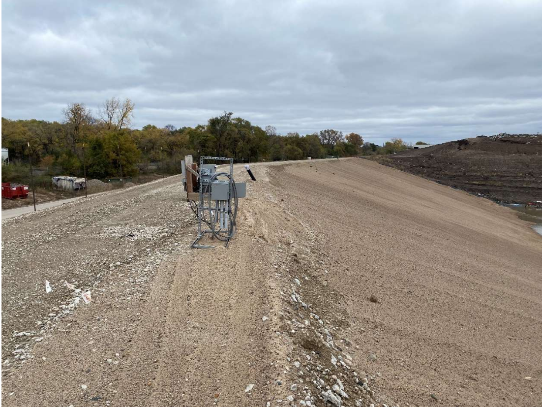
Location 13 – Cell 6, interior top of berm, looking north
