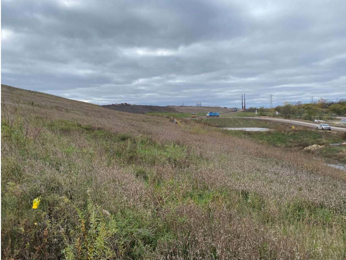
Location 18 – Cell 1 Toe of Waste Slope, looking southwest
