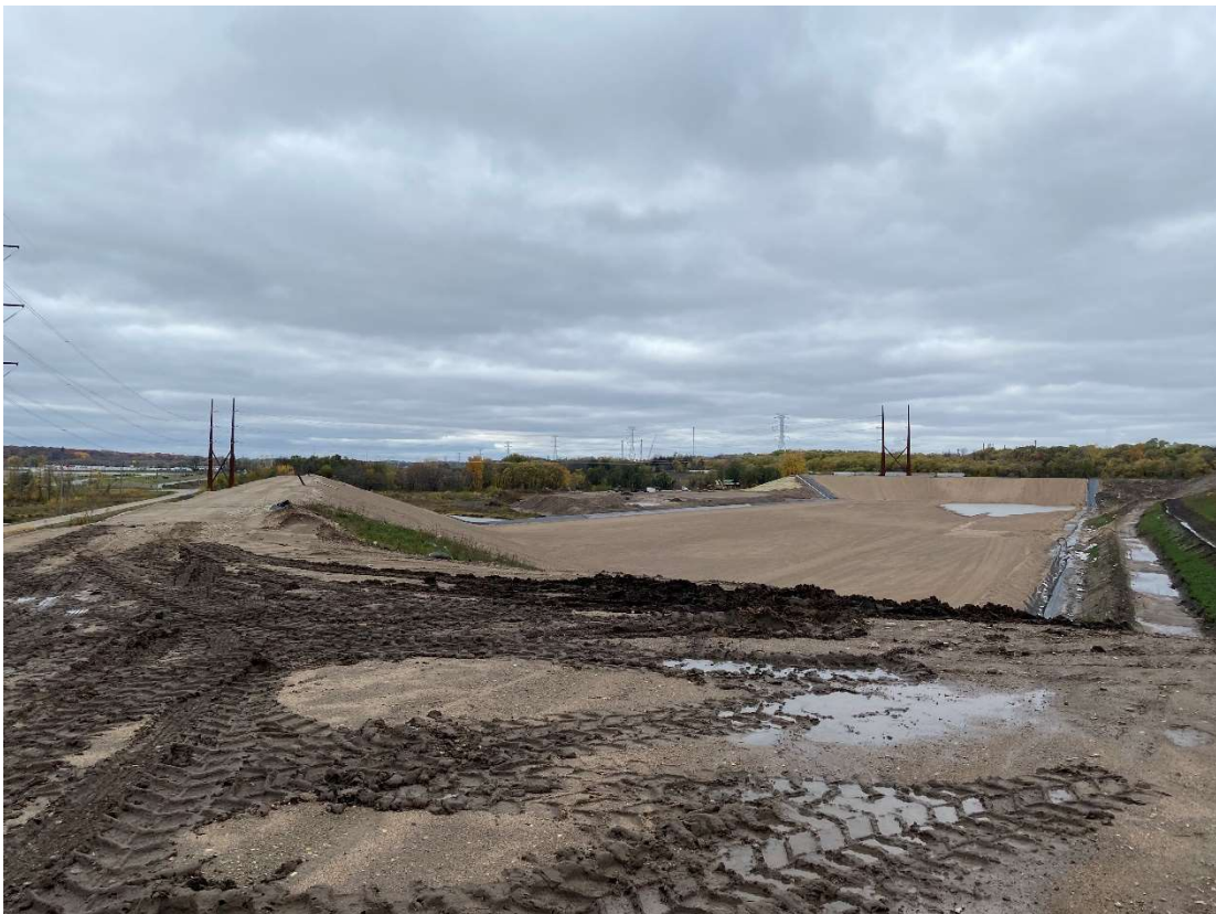
Location 7 – Cell 6, interior of southern landfill berm, looking west
