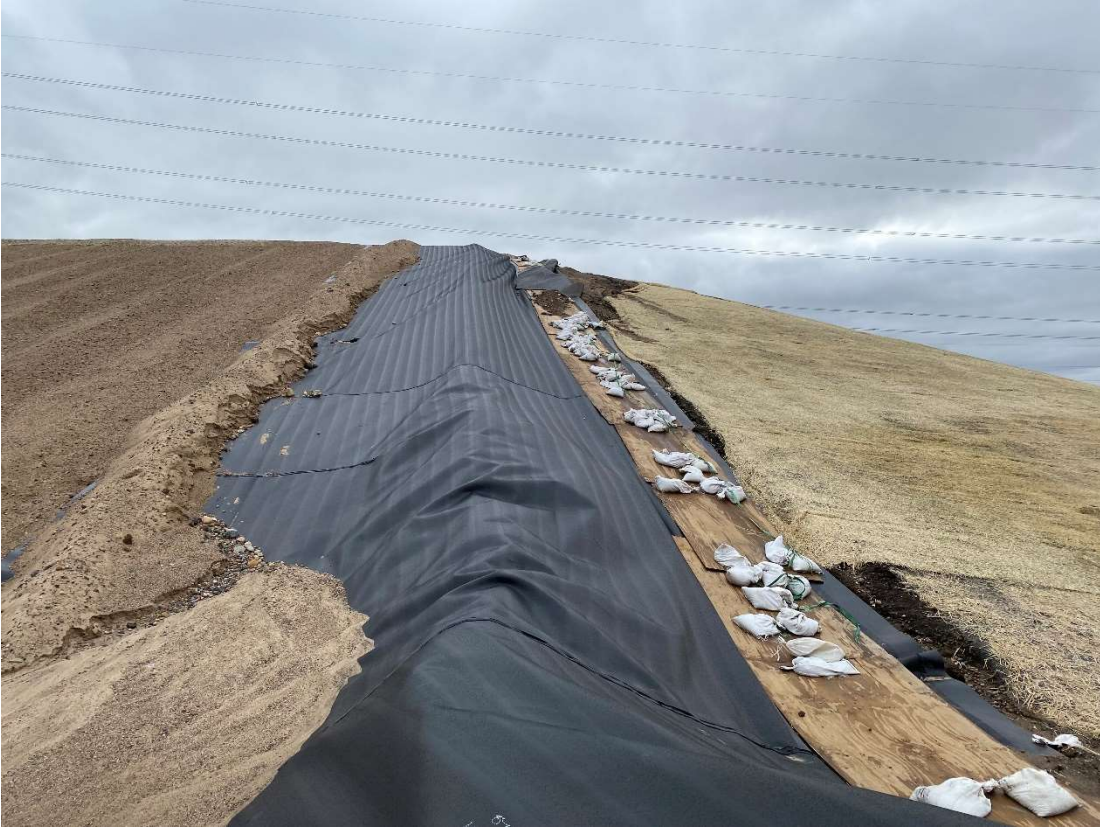
Location 9 – Cell 6, looking south along temporary phase construction berm
