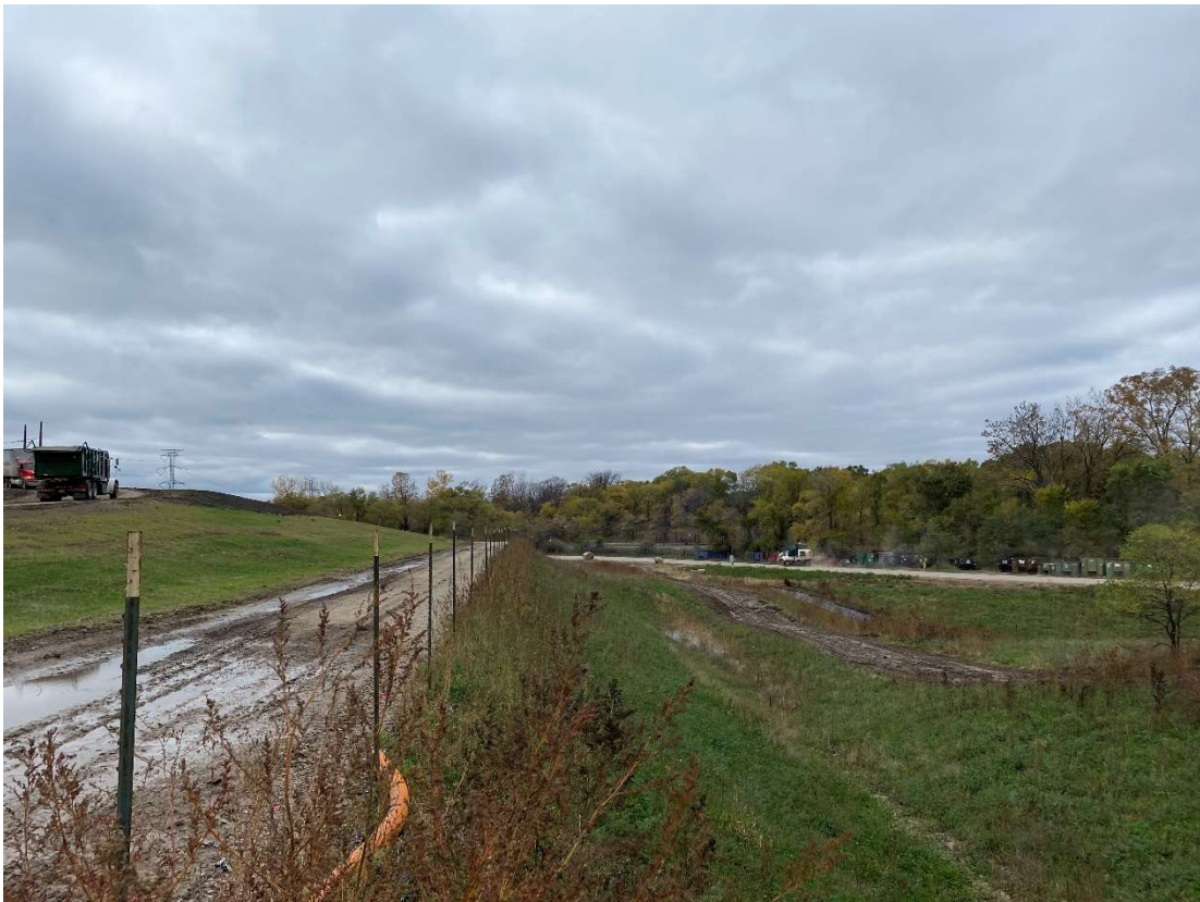
Location 17 – Cell 6 northern outer berm, looking southwest
