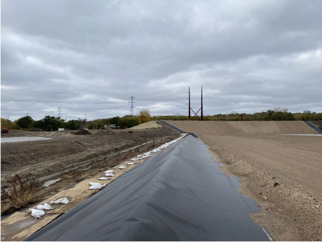
Location 10 – Cell 6, looking northwest along temporary phase construction berm
