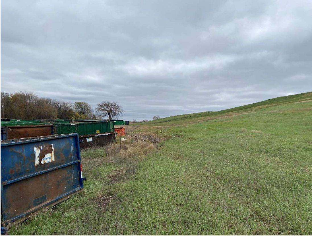
Location 2 – Looking Southeast, Cell 3A Anchor Trench and Northeastern Waste Slope
