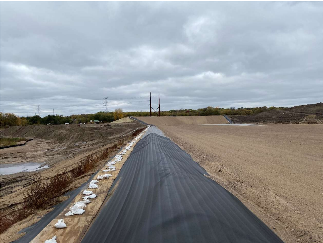
Location 9 – Cell 6, looking northwest along temporary phase construction berm
