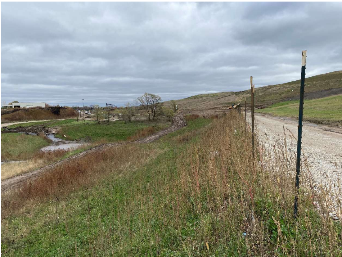
Location 16 – Cell 6 northern outer berm, looking northeast
