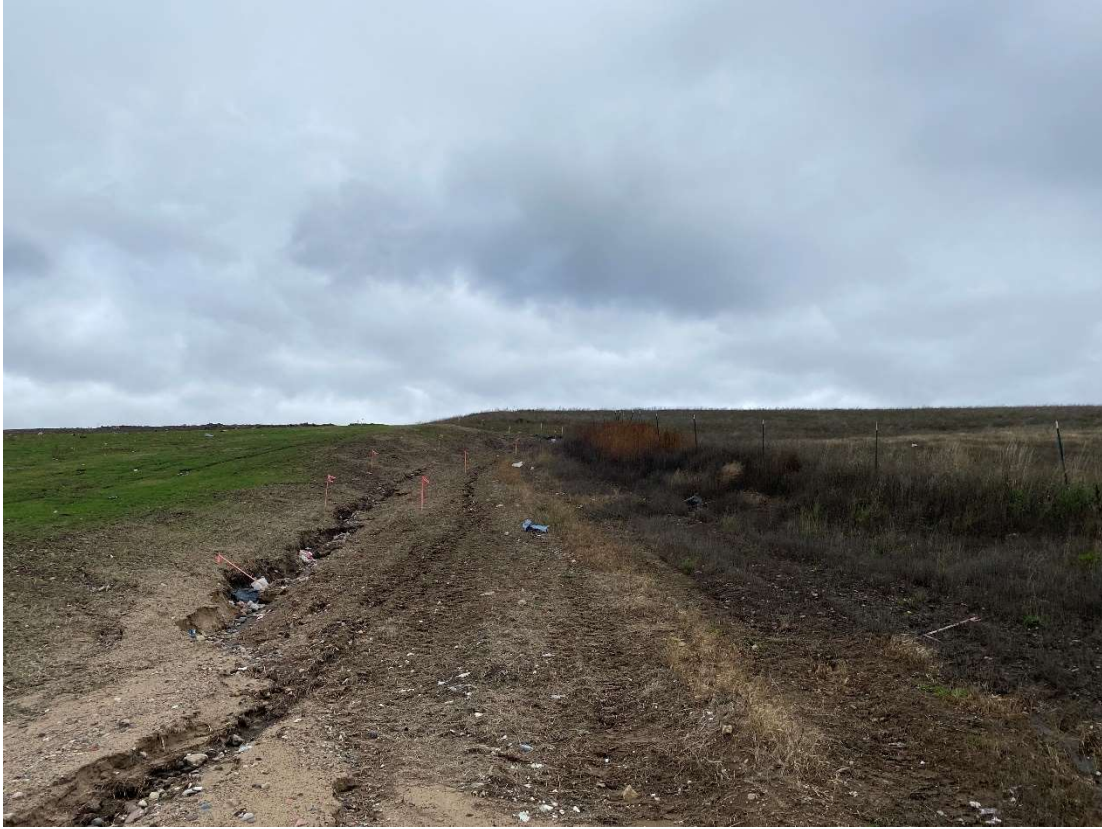
Location 6 – Cell 6, southeast corner, looking north at edge of overlay liner
