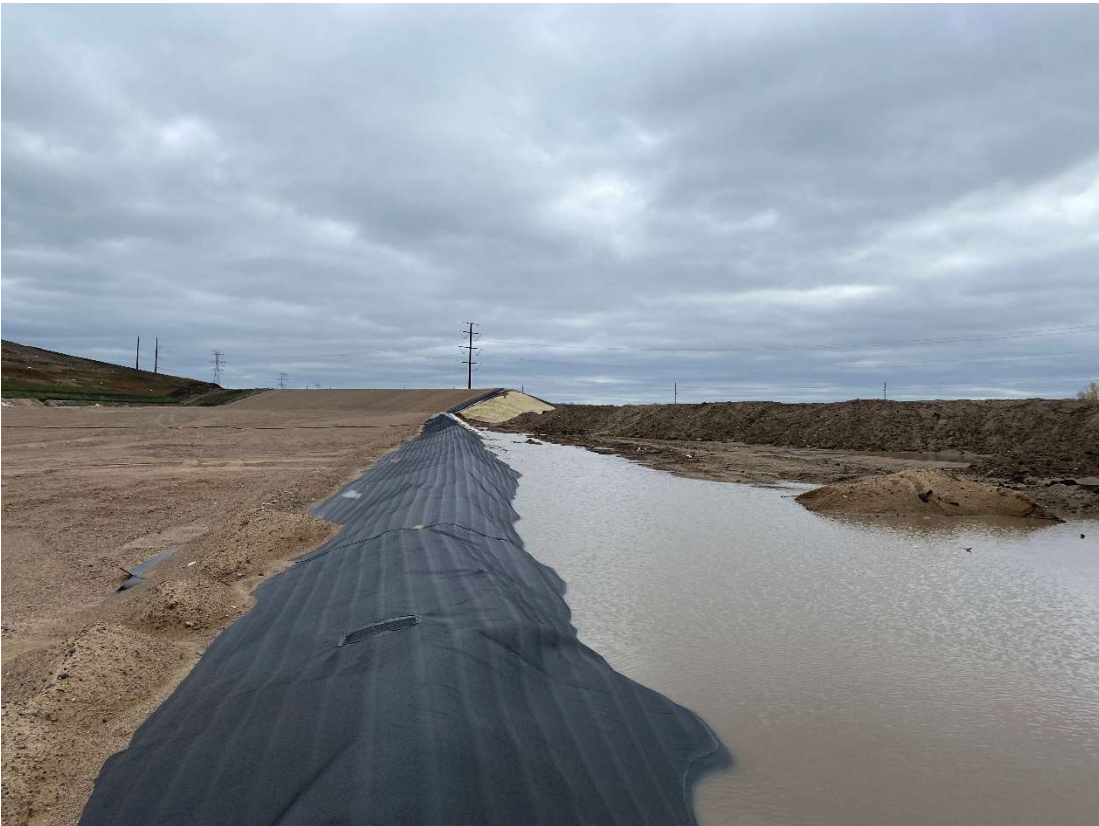
Location 11 – Cell 6, looking southeast along temporary phase construction berm
