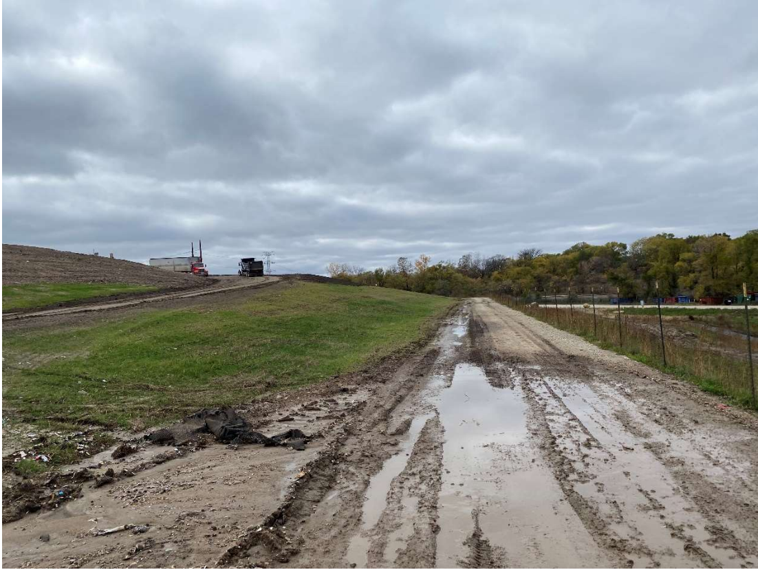
Location 17 – Cell 6 northern top of berm, looking southwest
