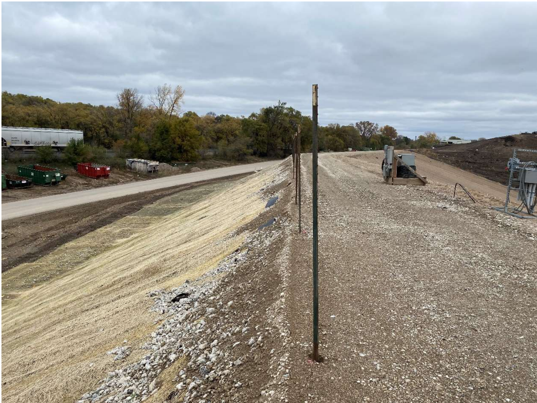
Location 13 – Cell 6, exterior top of berm, looking north
