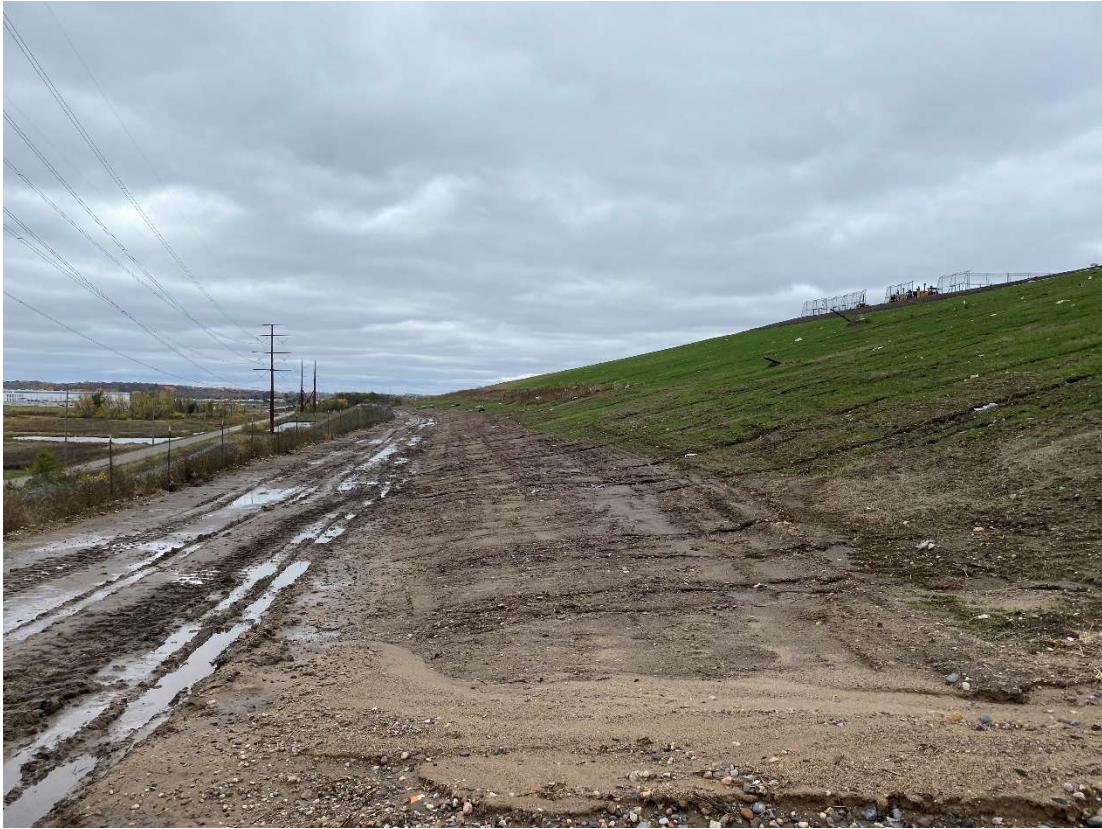
Location 6 – Cell 6 southeast corner, toe of southern waste slope, looking west
