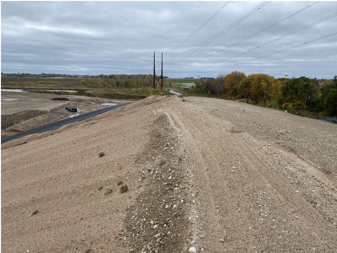
Location 13 – Cell 6, interior top of berm, looking south
