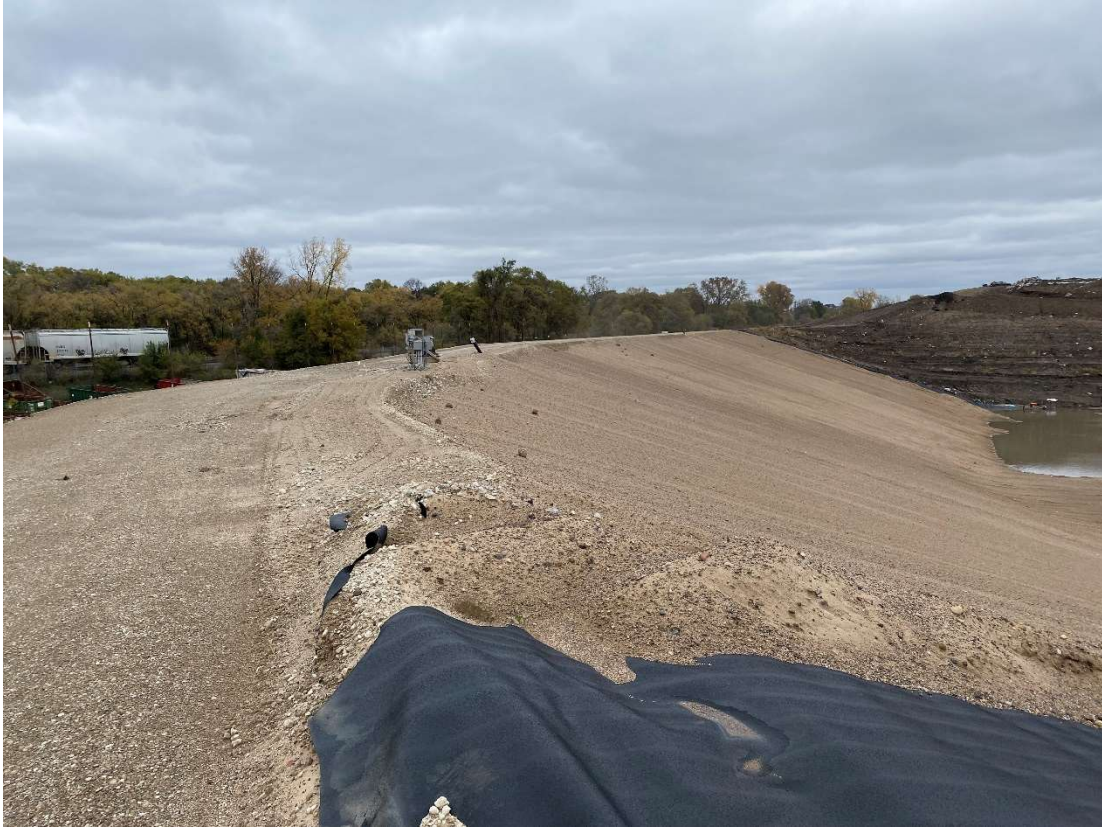
Location 12 – Cell 6, interior top of berm, looking north
