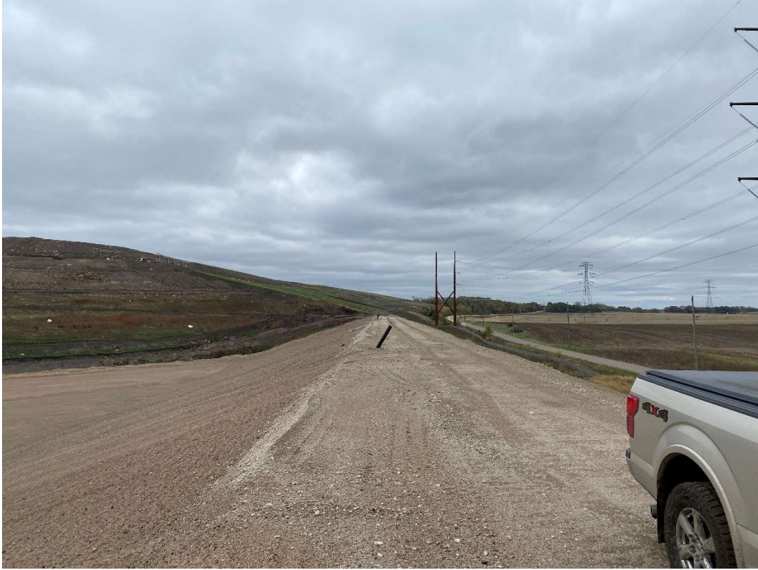
Location 8 – Cell 6, interior of southern landfill berm, looking west
