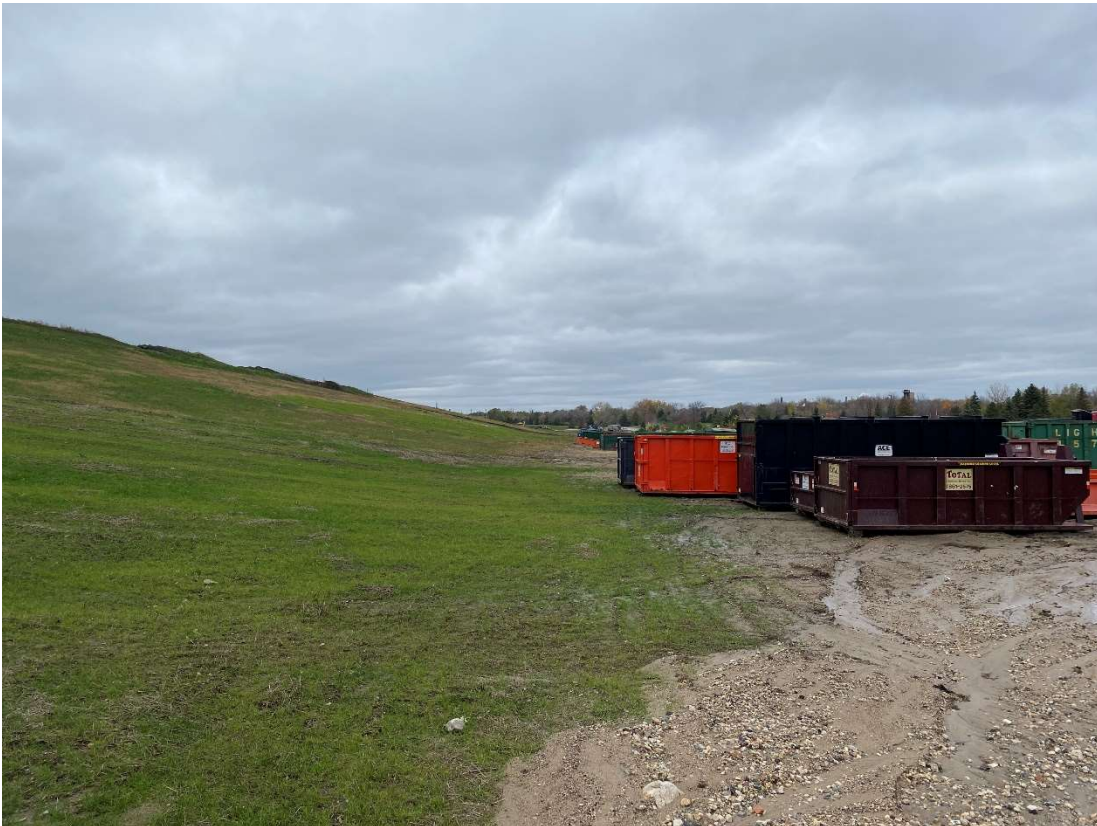
Location 3 – Looking Northwest, Cell 3A Anchor Trench and Northeastern Waste Slope
