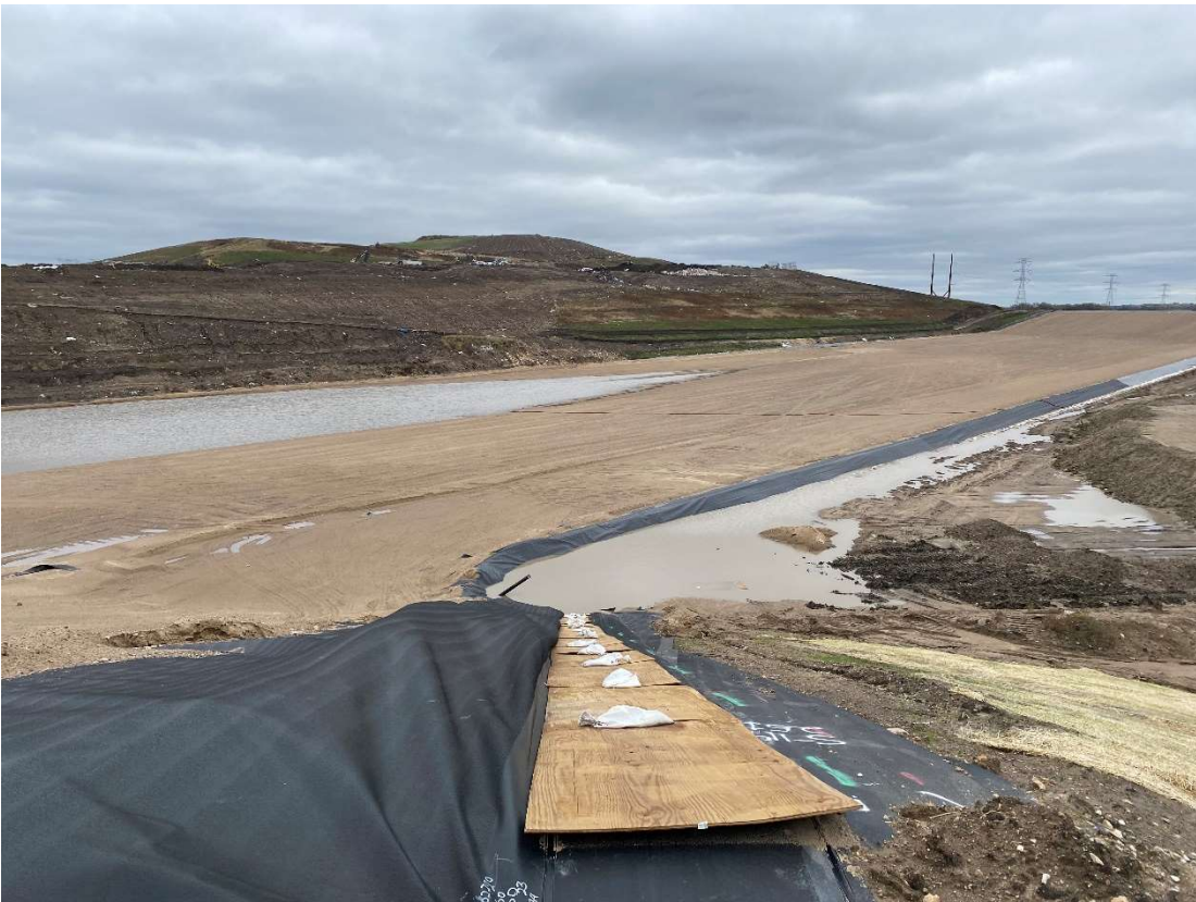
Location 12 – Cell 6, looking east along temporary phase construction berm
