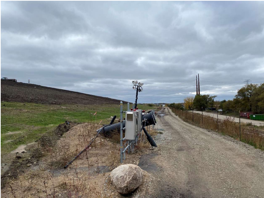
Location 16 – Cell 6 northwestern top of berm, looking southwest
