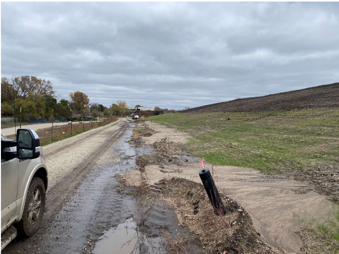
Location 15 – Cell 6 northwestern toe of waste slope, looking northeast
