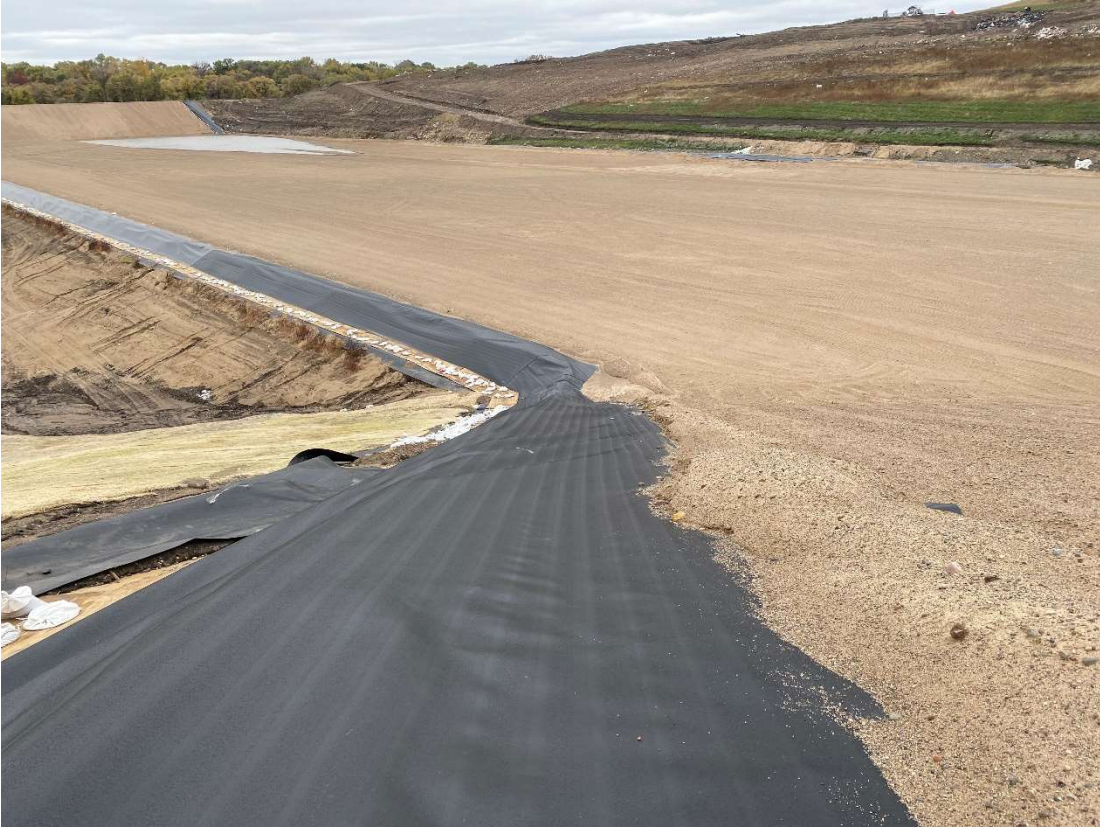
Location 8 – Cell 6, looking north along temporary phase construction berm
