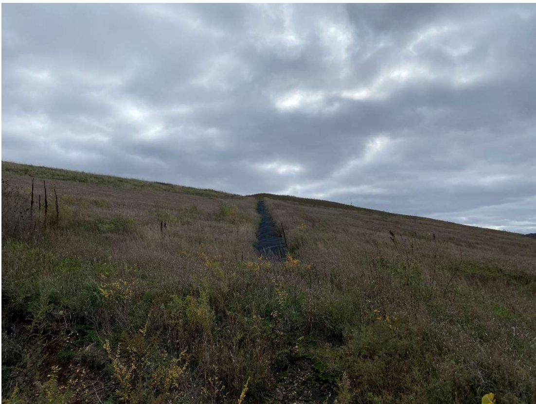
Location 18 – Cell 1 edge of cap, looking south
