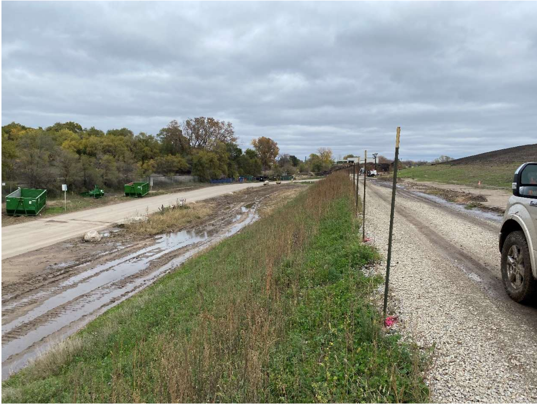
Location 15 – Cell 6 northwestern outer berm, looking northeast
