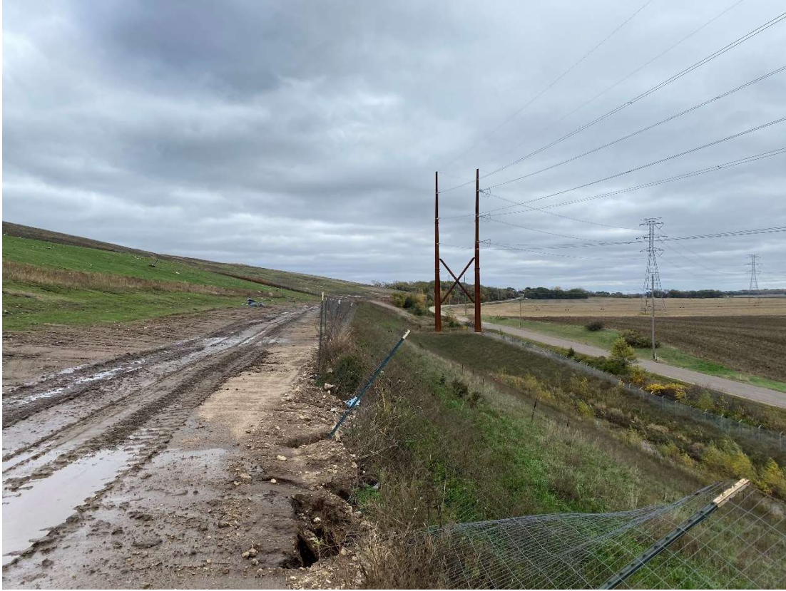
Location 7 – Cell 6, southern outer berm, looking east
