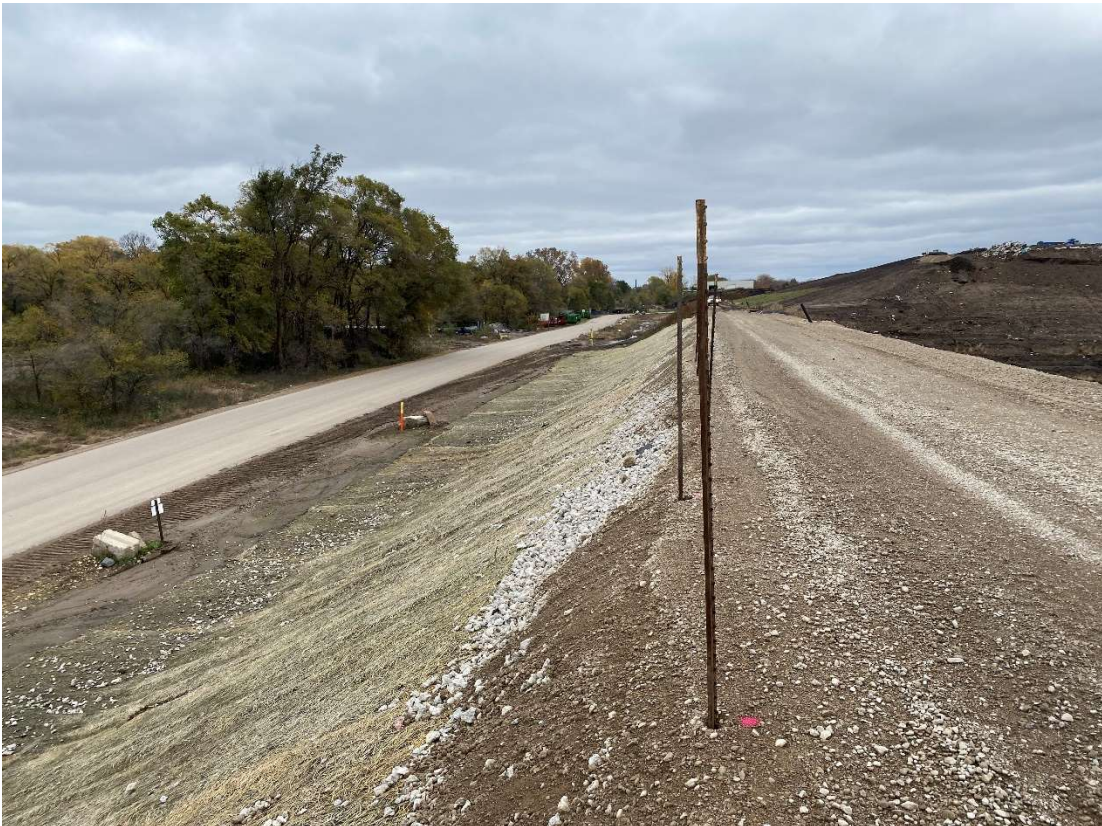
Location 14 – Cell 6, exterior top of berm, looking north
