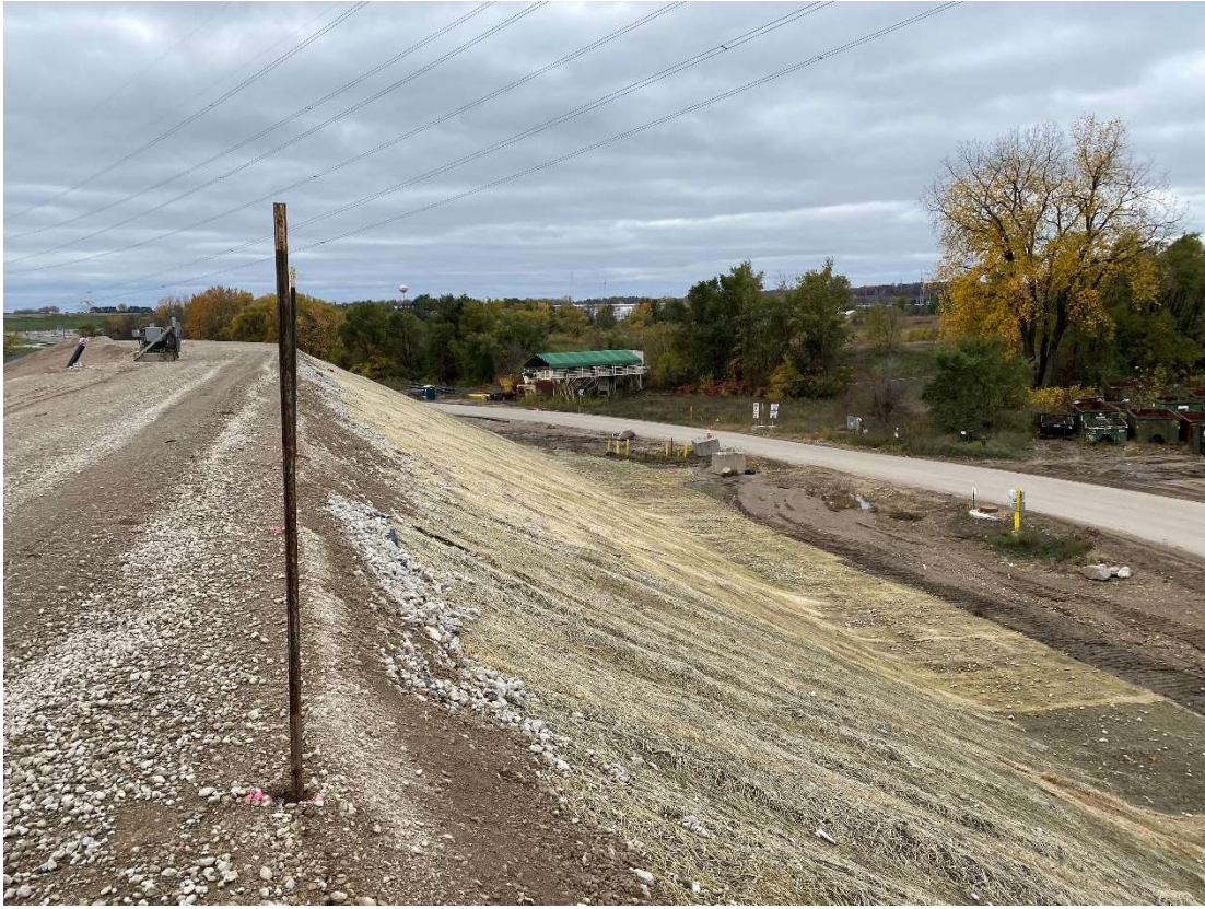
Location 14 – Cell 6, exterior top of berm, looking south
