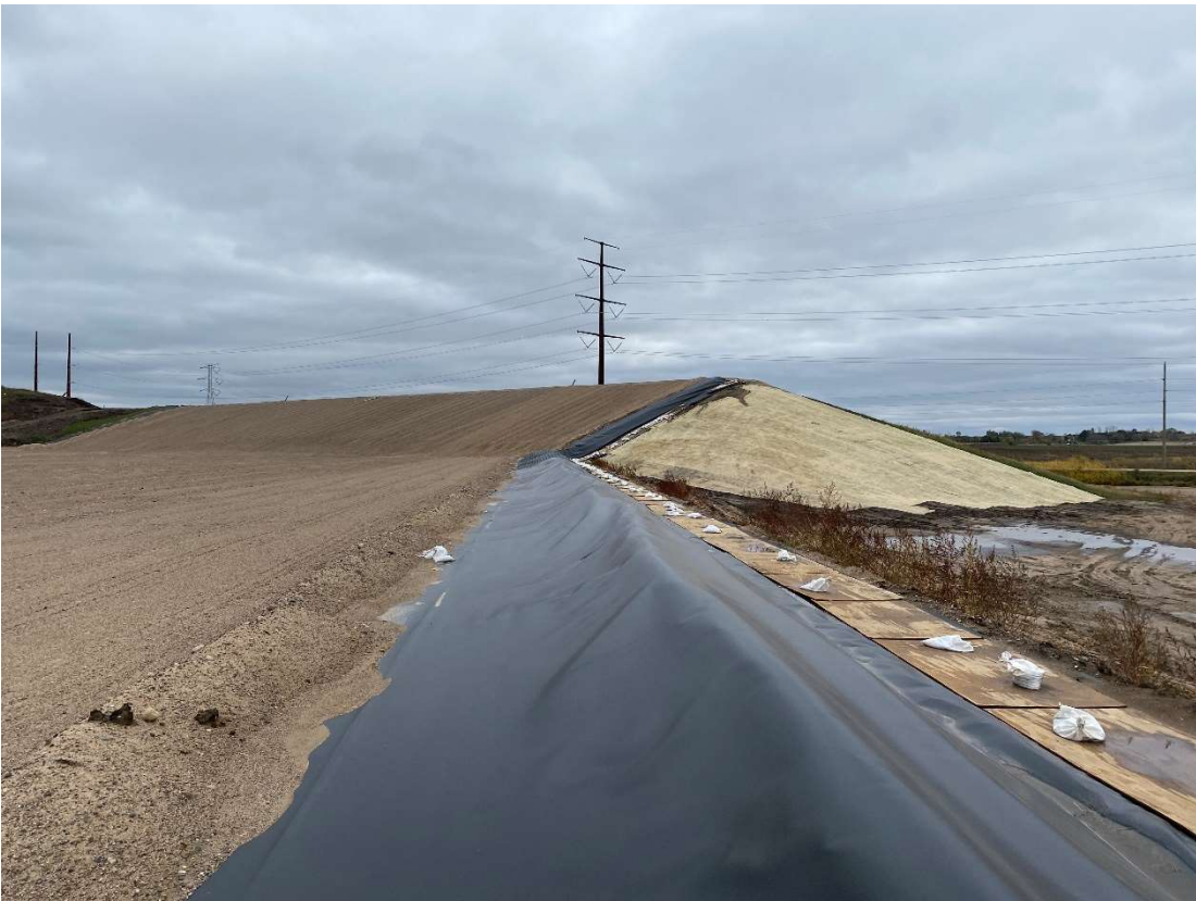
Location 10 – Cell 6, looking southeast along temporary phase construction berm
