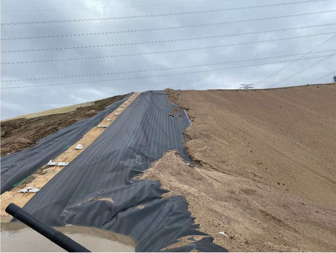
Location 11 – Cell 6, looking west along temporary phase construction berm
